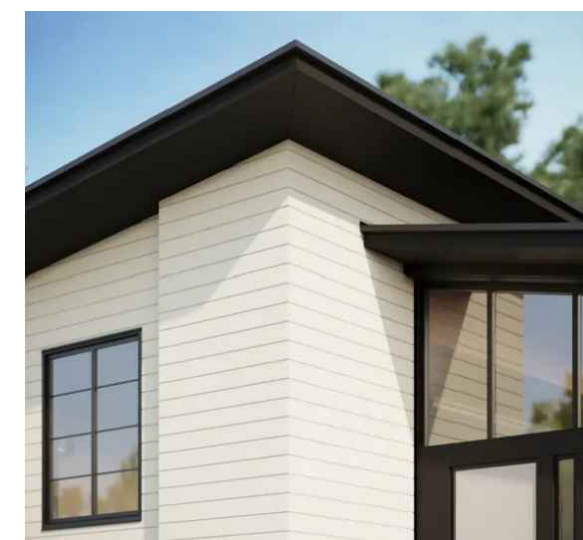
(M2) SIDING: HARDI PANEL V-GROOVE ARTISAN BOARD
